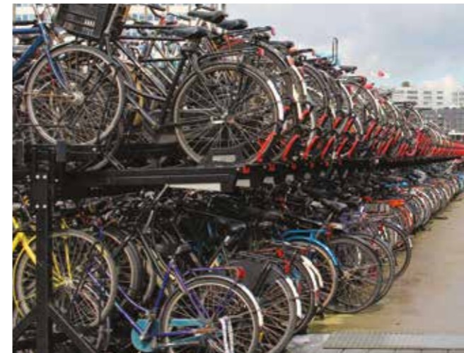
Two-tier stand Adds capacity by stacking bikes but should only be used for larger scale cycle parking and ideally be under cover (must meet criteria laid out in Section 4.2 of this document). Should not be used to provide 100% of cycle parking as they are not compatible with non-standard cycles and some users struggle to use them.
