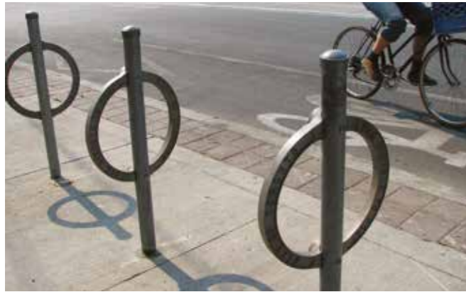
Cyclehoop Provides a good alternative in situations where a Sheffield stand or equivalent is not feasible - provides less support for the bike but can be clamped to an existing post.
