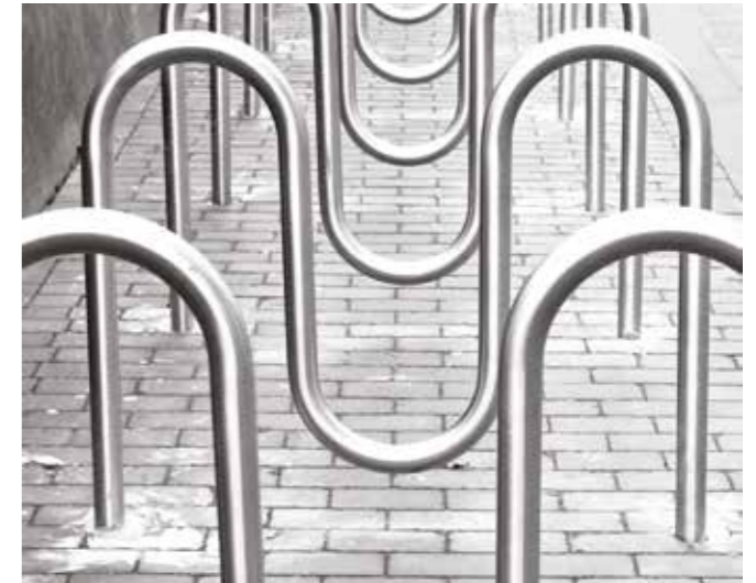
Camden 'M' stand Parks 2 bicycles and is a variation of the Sheffield stand and encourages locking the bicycle frame in two places.
