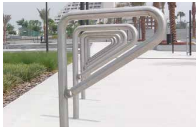
P-stand Hard to use for two bikes side by side as it provides only one area for locking wheels and frame. Can be used however in areas of low demand.
