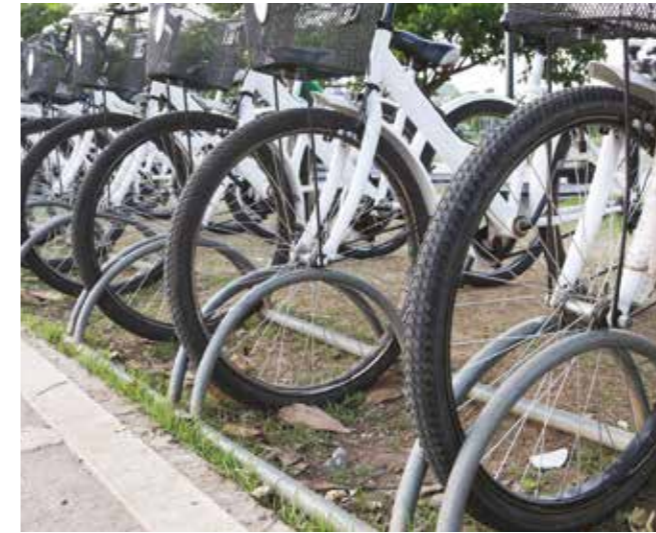
Wheel racks These must be avoided as they provide no locking points for a bicycle frame and provide no support. They can also damage bicycle wheels.
